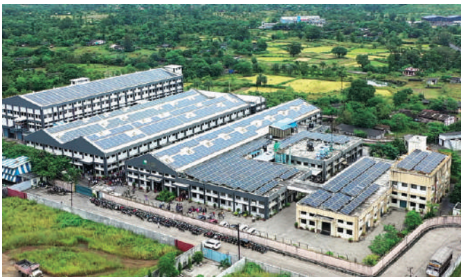
Massive State-of-the-art manufacturing facility with solar panels & RWH, in Palghar
